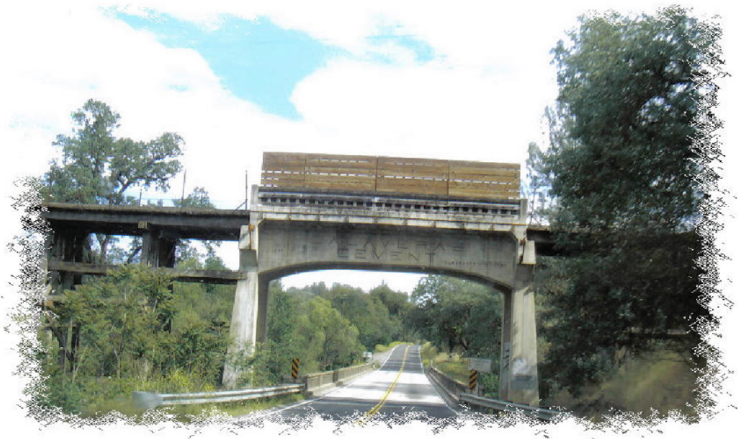
Calaveras Cement Bridge
